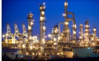
Pressure Boundary Bolted Joints
